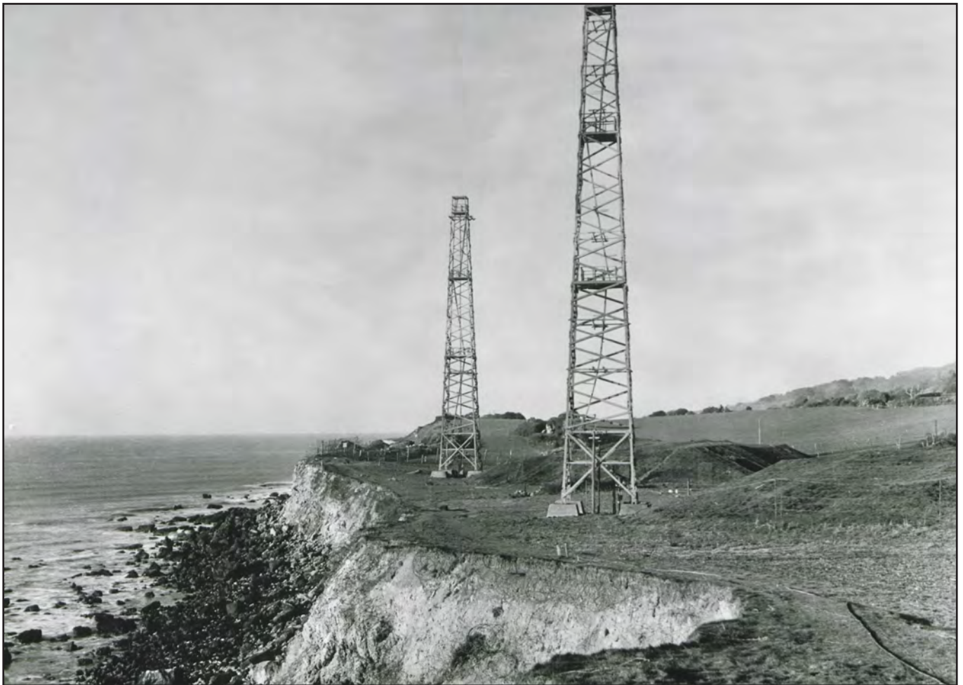
Figure 24. Radar station on the UK coast. WW2 saw the first use of radar in meteorology.
