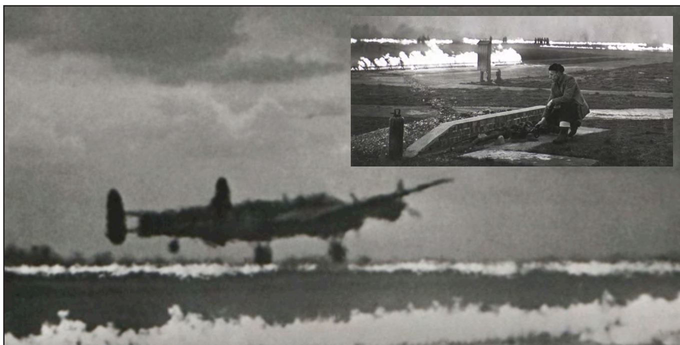
Figure 13. An aircraft using an airfield that has been cleared of fog using Fog Investigation and Dispersal Operation (FIDO). The ring of flames around the airfield is formed of burning petroleum, the heat from which was used to disperse the fog.
