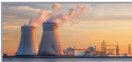
Factories and power stations
