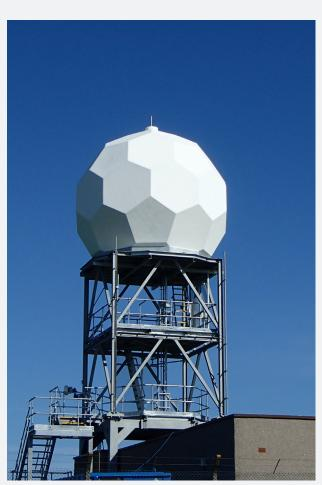
Radars have small devices in them called receivers. A receiver 'listens' to the pulses transmitted back to the radar. From these, we are then able to work out how far away the precipitation is, how heavy it is and even what type of precipitation it is likely to be.
